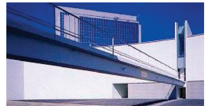
Photo 7 技術研究所の連絡橋 (1993年竣工) (Fc = 100N/mm 2 , スパン = 40m, 桁高 = 1m) Pedestrian bridge in the research institute (Fc = 100N/mm 2 , span = 40m, depth = 1m)
