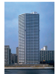
Photo 1 セーラ小松川10号棟 ( F_c = 48\text{N/mm}^2 , 33F) An example of high-rise RC buildings in 1980s
