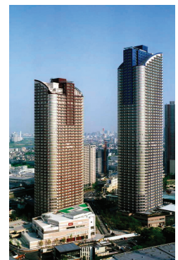
Photo 2 パークシティ武蔵小杉 ( F_c = 150\text{N/mm}^2 , 59F) An example of present high-rise RC buildings
