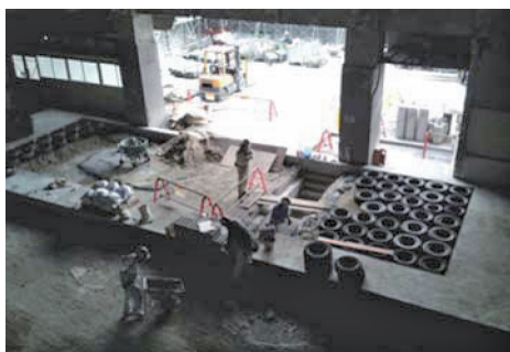
Photo 4 タイヤの敷設状況 Laying of car tires
