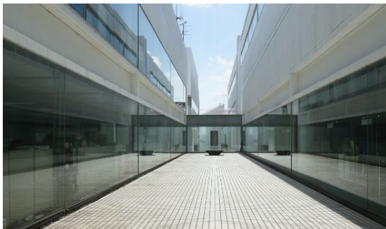
Photo 1 Workplace and courtyard before renovation
