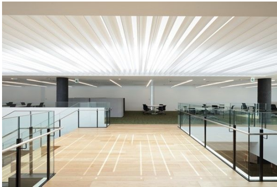
Photo 20 Efficient use of natural energy with Y-shaped electric controlled louvers
