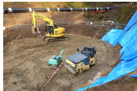
(b) Completion of installation of protective embankment
