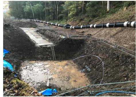
(a) Completion of river diversion and protective embankment excavation
