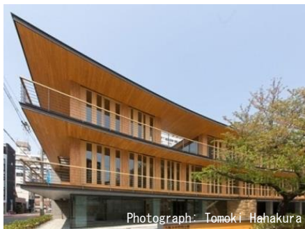
Photo 2.1 Osaka Timber Association Building
