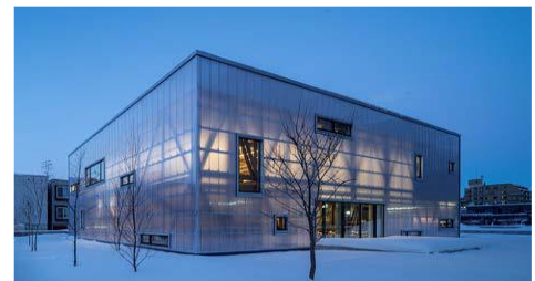
Photo 5.2 Building exterior (viewed from the southwest)
