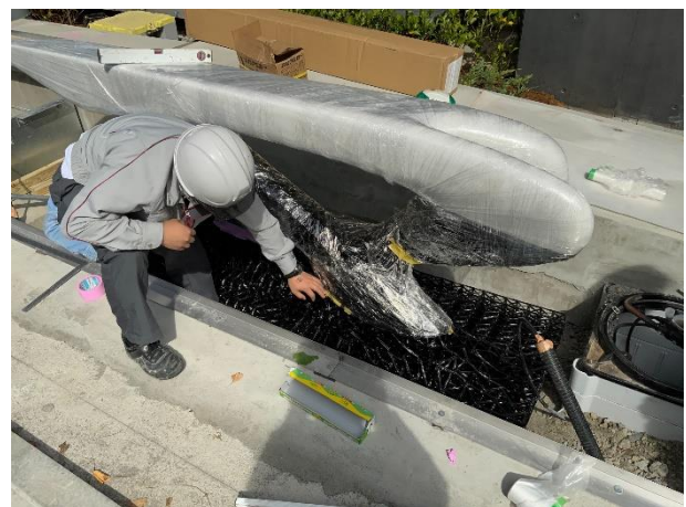
Photo 4.4 Installation status on site
