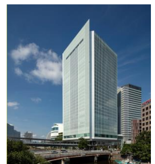
Photo 5.1 Exterior view of the building (Photographed by Shigeo Ogawa)
